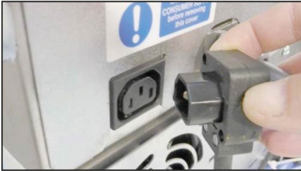
Figure 46: Plugging in the condenser unit
